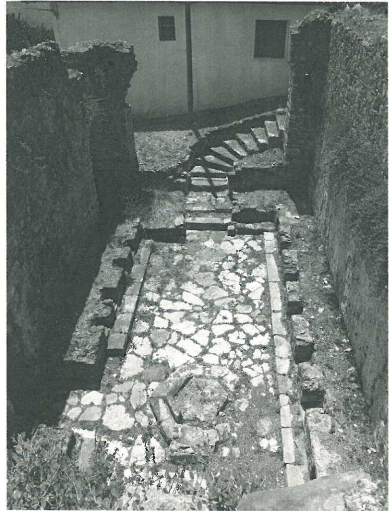
Fig. 6. Entrance to the monumental bath building in the külliye complex with changing area and hexagonal fountain (seen from the north).
